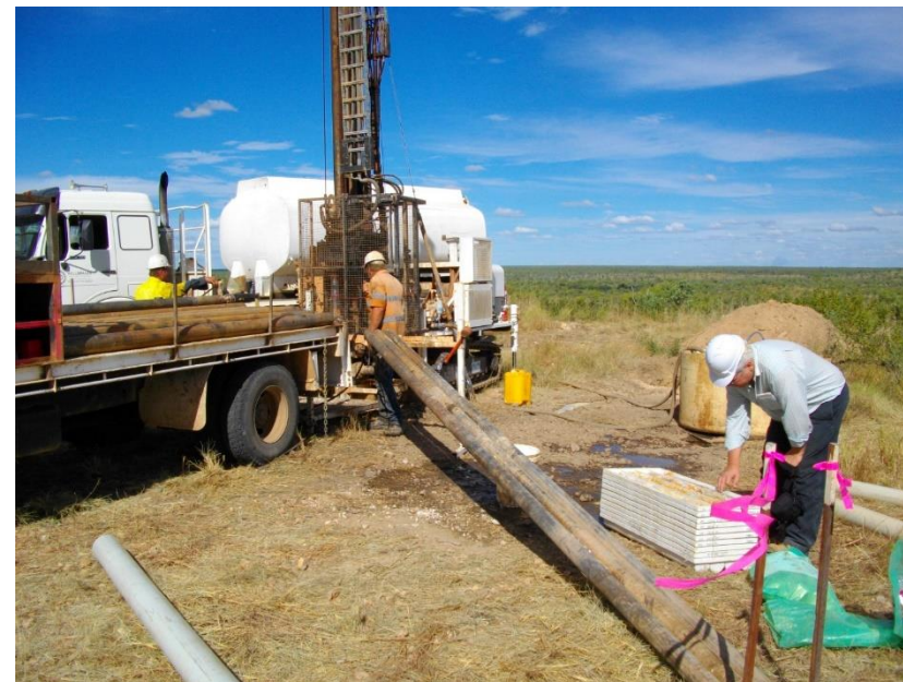
Core Drilling at Highland Plains
