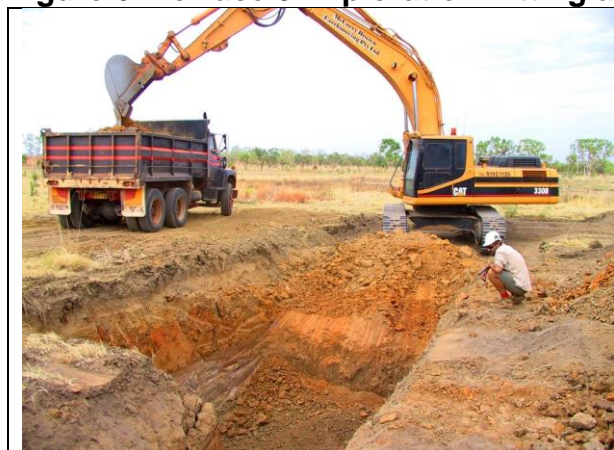
Exploration pitting at Blina using an excavator
