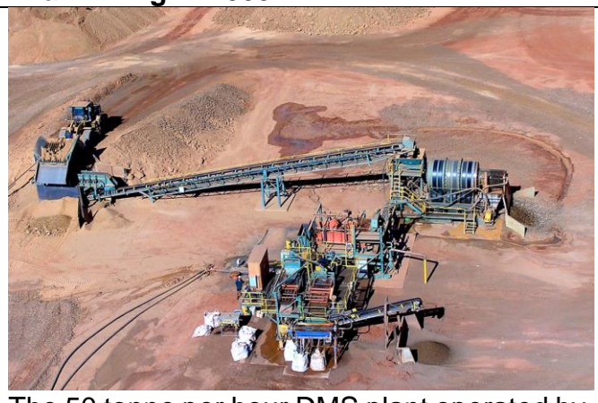
The 50 tonne per hour DMS plant operated by Blina Diamonds NL in 2005
