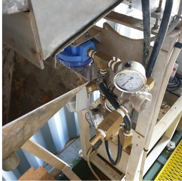
New fittings have been installed throughout
