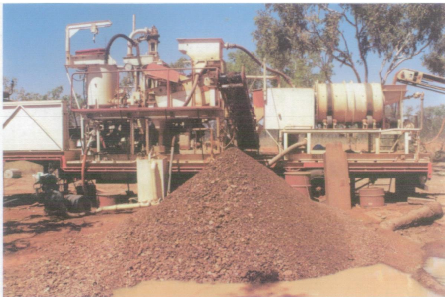
Diamond Ventures NL Plant operating in 2001 on what is now POZ Mining Lease M04/467
