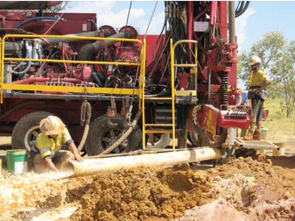
Water Bore Drilling at Highland Plains
